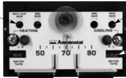
Heating & Cooling Wall Thermostat (Cover Removed)
